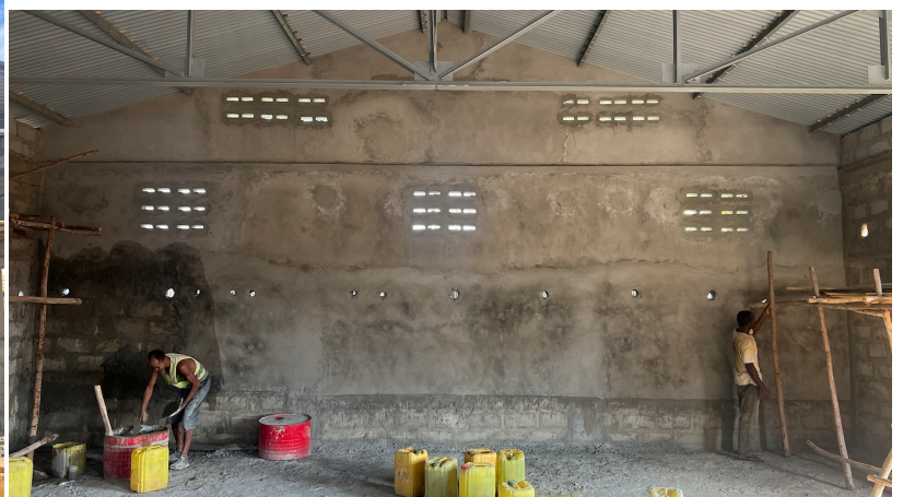
Stuccoing the cinderblock walls of the church building
